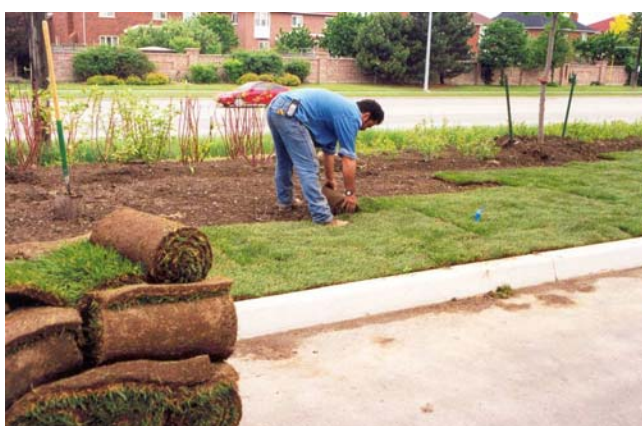
Installing sod on Boulevards.
