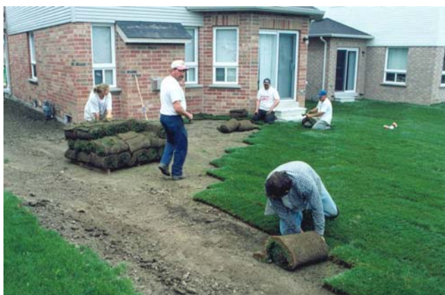
Installing sod in a brick laying method.
