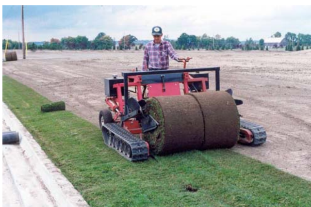
Installing Big Rolls with a special laying machine.
