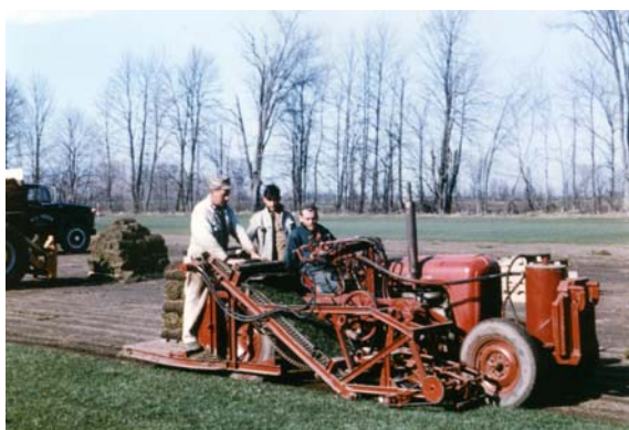
This was the first prototype Sod Harvester (Roll) made by Gerry Brouwer in May 1966. It only cut sod and brought it up the conveyor where one man rolled it up, another stacked it on the pallet and the driver.
