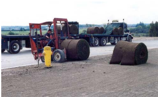
Unloading and placing Big Rolls ready to install.
